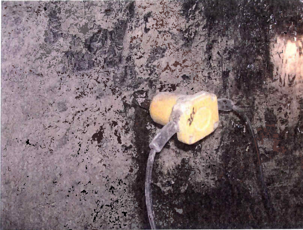
Figure 6: Example of geophone installed in coal rib. A hole is drilled into the rib and the spike on the geophone is pushed into the hole until a snug fit is obtained.
